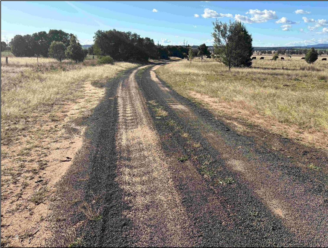
Photo 7: Site access, west end, north orientation. Imported gravel over a land formed surface. Photo: D. Wall, 2025
